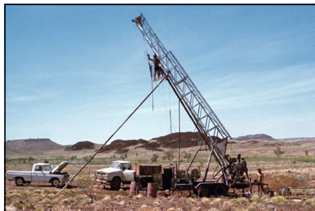
Figure 34. Drilling to prove nickel reserves at Whundo.
