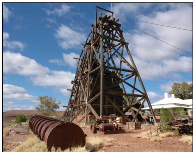
Figure 12. Shaft headgear at the Sons of Gwalia gold mine.
